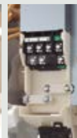
Bigger working space for wiring connection.
